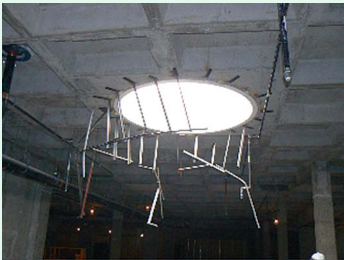
This skylight is where the old McHenry Library's signature spiral staircase was located. Though loved by many it was a fire hazard and had to go.
